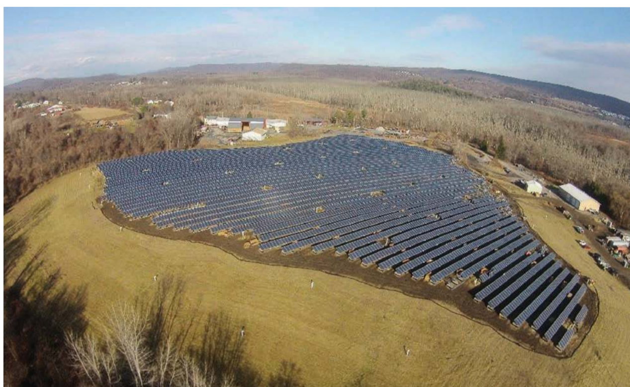
A 1.3MW solar array installed by the author's company, BQ Energy, on a 25 acre municipal landfill site in Patterson, NY.
